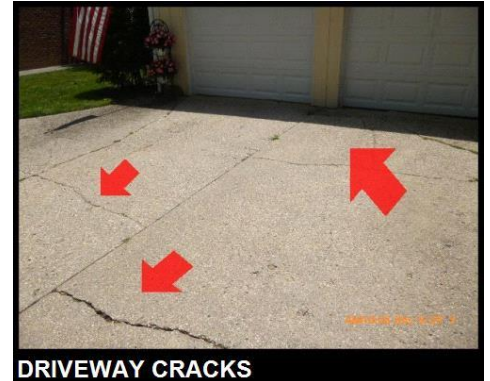
DRIVEWAY CRACKS
