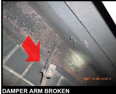
DAMPER ARM BROKEN
