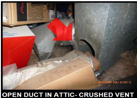
OPEN DUCT IN ATTIC- CRUSHED VENT
