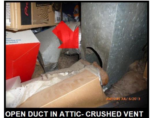
OPEN DUCT IN ATTIC- CRUSHED VENT
