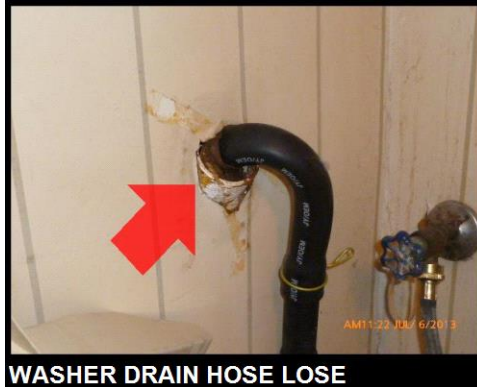
WASHER DRAIN HOSE LOSE
