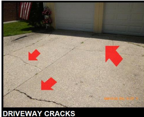
DRIVEWAY CRACKS
