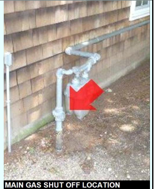
MAIN GAS SHUT OFF LOCATION
